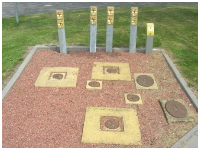
Figure 14. Electricity site in public space, Zierikzee, NL (photo by Charles Forceville, 2007).
